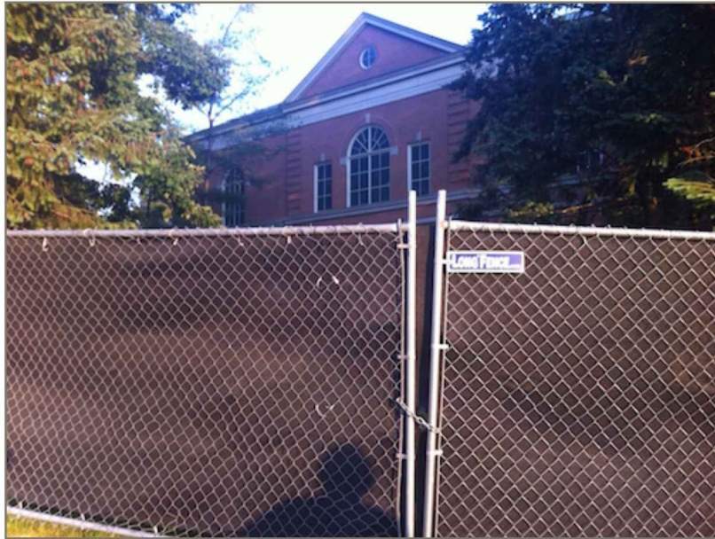
THE MARRIOTT HOTEL IN CHANTILLY, VIRGINIA PROTECTED BY A TEMPORARY PRIVACY AND SECURITY FENCE SET UP FOR THE 2012 MEETING.
