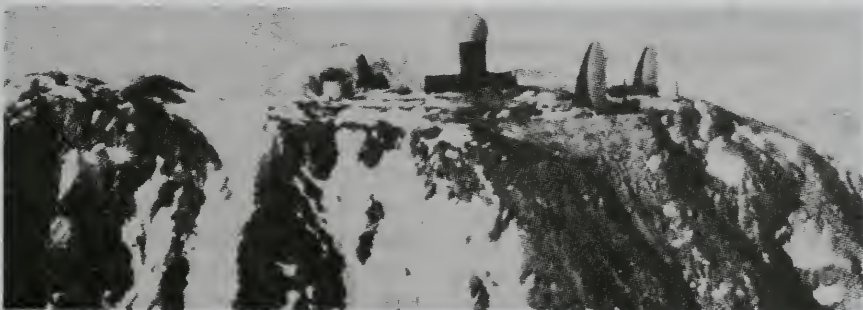
Washington taught that preparation for war was a necessary means of preserving peace. This radar station on Greenland's eastern coast is one of America's Distant Early Warning Line installations in the Arctic.
